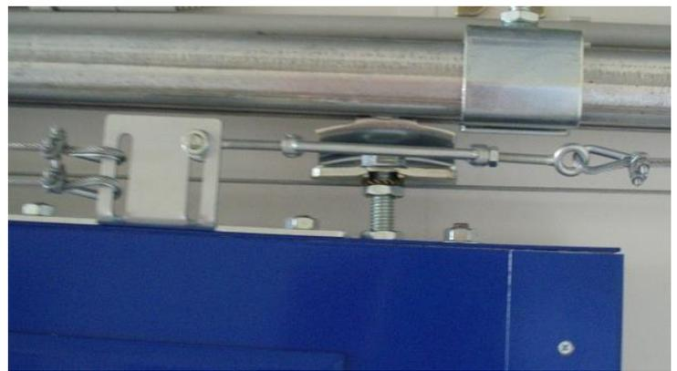
Door pull with screw turnbuckle
