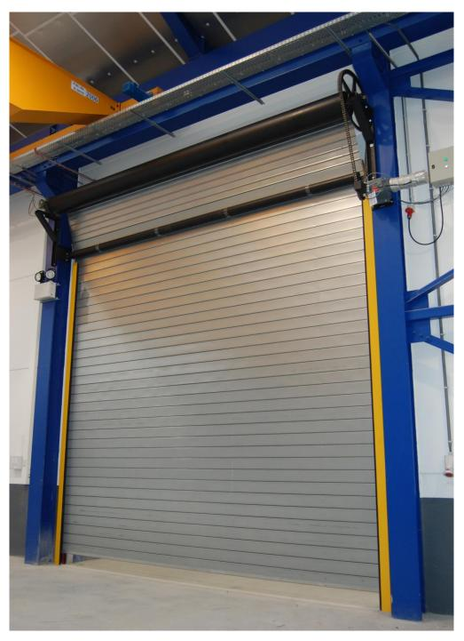
The rolling fire shutter is designed to separate two fire areas automatically without human intervention and for a defined period of time, has created fire barrier to prevent or limit the spread of fire. The fire gates are not determined, due to their weight, for frequent use as the ordinary gates. Their primary function is closing in case of fire. Recommended number of opening/ closing is max 5x/ hour.
